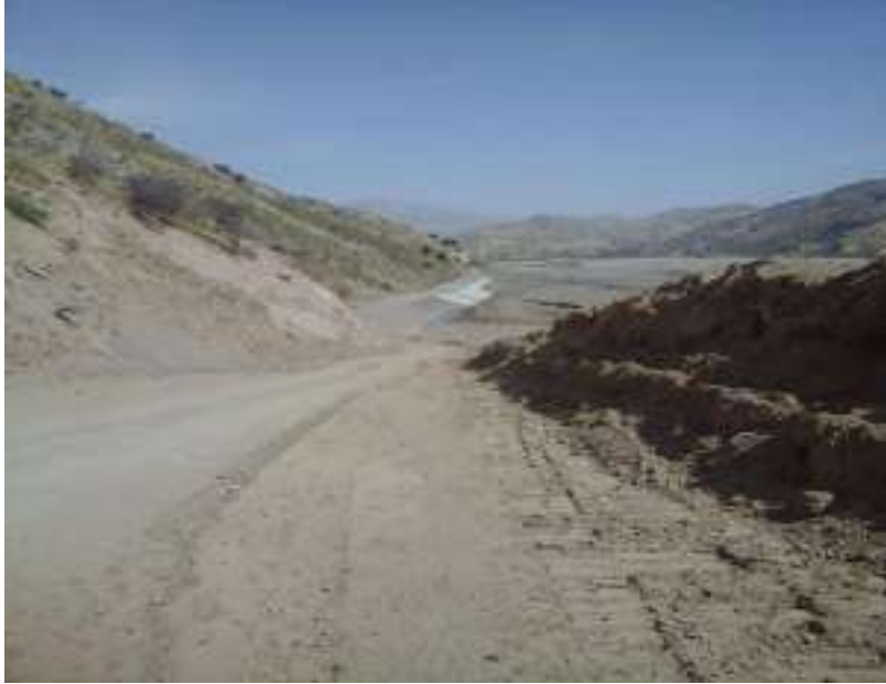
Figure 5 – Existing Road at km 2.88
