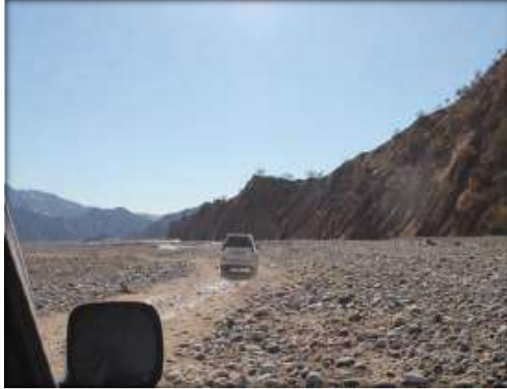
Figure 7 – Existing Road at km 47
